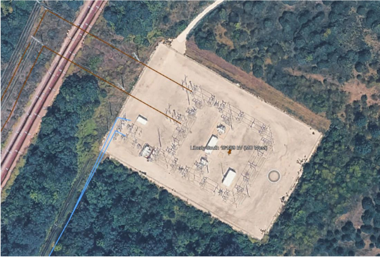
Figure 1 – Liberty South 161/69kV Substation
